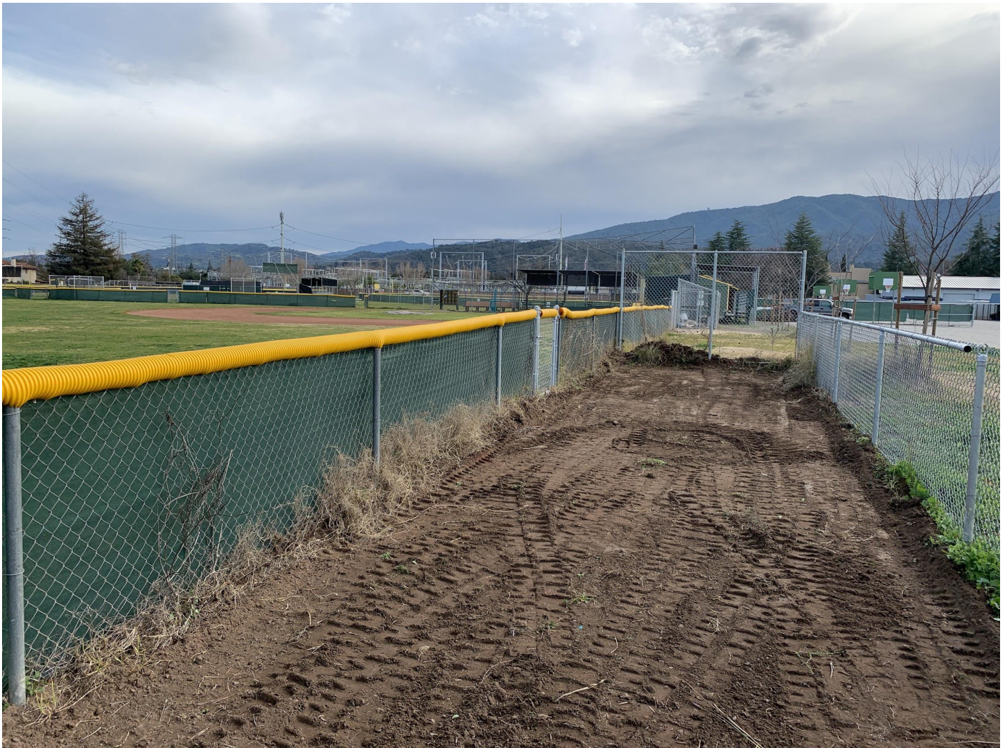
Starting Bullpen Grading and Repairs
